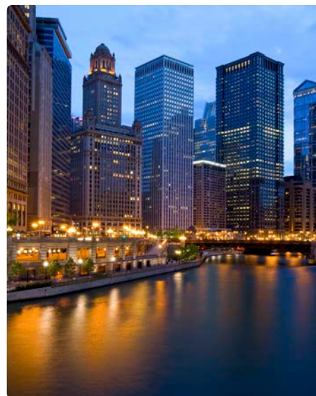
In 2013, ComEd made great progress toward its vision of being a 21st century utility that delivers exceptional value and service to customers.
